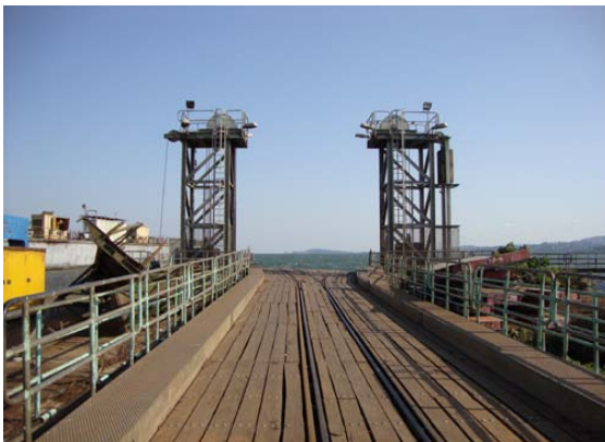
Figure 7-5 Wagon-Ferry Ramp at Port Bell
