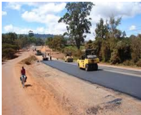
Figure 6-4 Road Construction Activity
