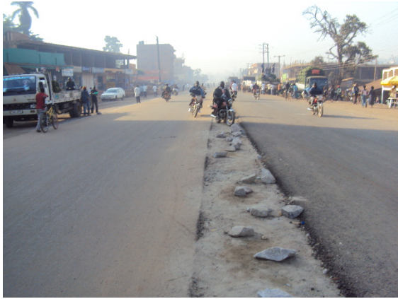
Fig. 3: New Road under Construction in Kampala
