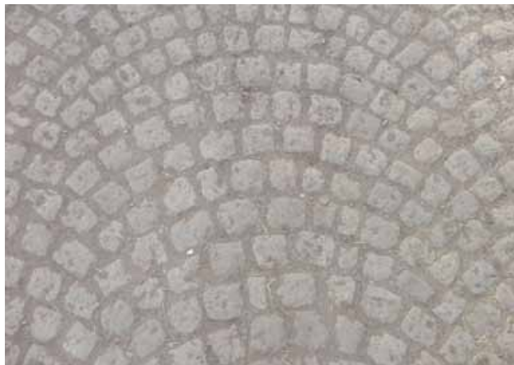
Photo 7-1: Example of Cobble Stone surfacing
