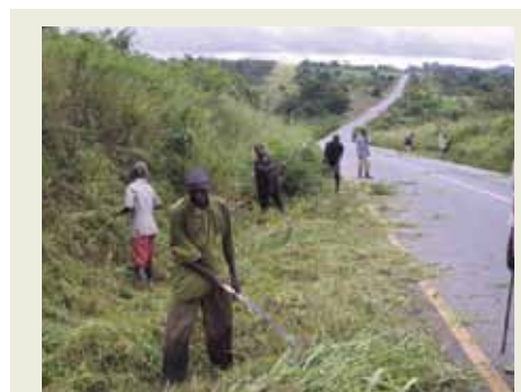
Grass cutting—a typical, labour-based routine maintenance activity.
