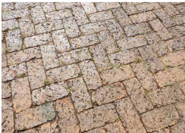
Photo 7-2: Example of burnt Clay Brick surfacing (Herringbone pattern)
