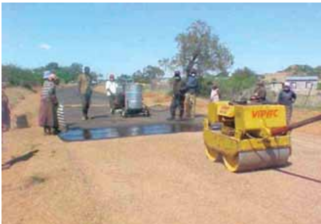
Compaction of Natural Sand Sealed Section
