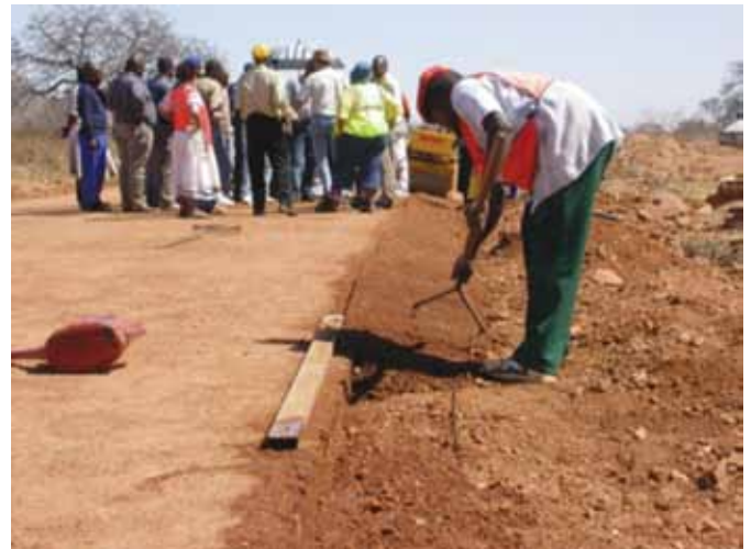
Edge Cladding of Based Layer
