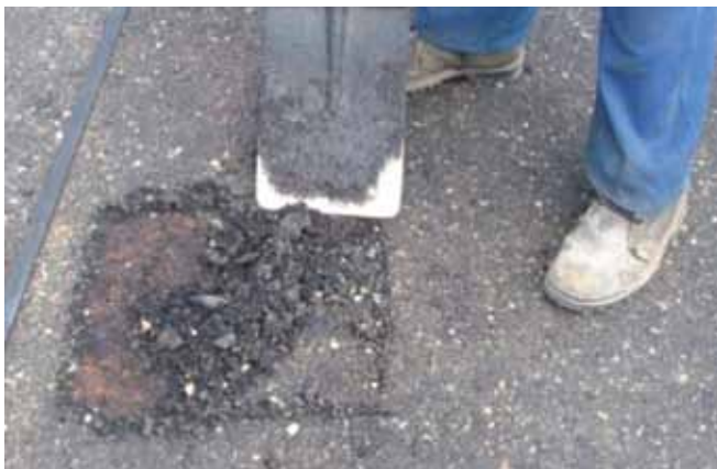
Removal of old material
