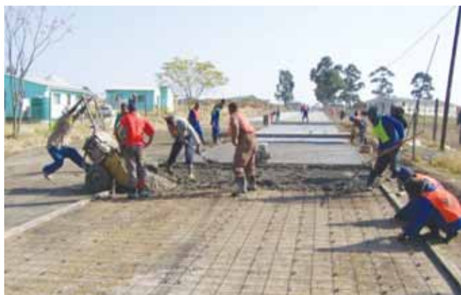
Laying of ultra-thin concrete
