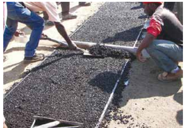
Screeding the asphalt
