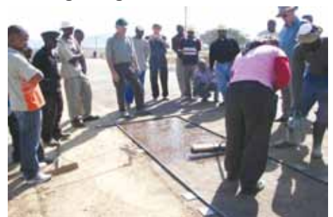
Application of tack coat
