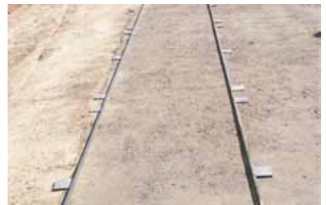
Placing the guard rails
