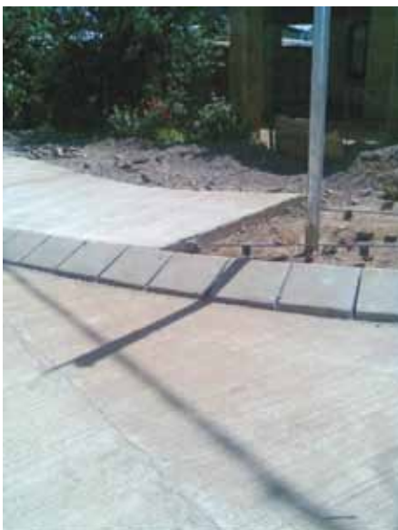
Completed UTRCP sections
