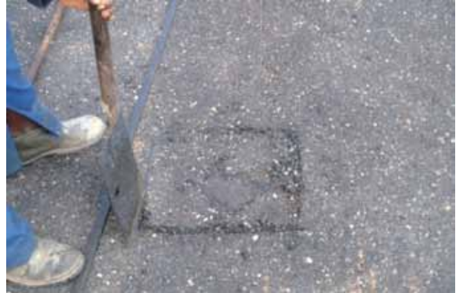
Trim the pothole area
