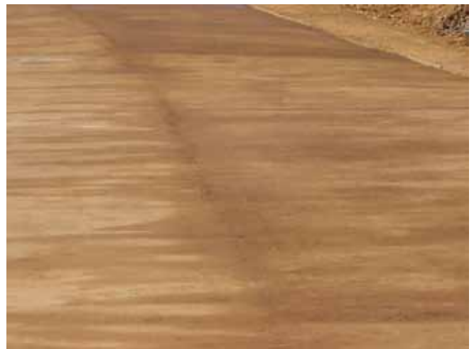
Compacted stabilized base
