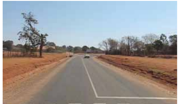
A completed Otta Seal section
