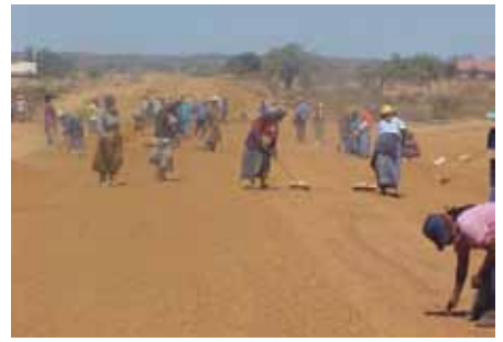
Sieving of natural aggregates at the borrow pit
