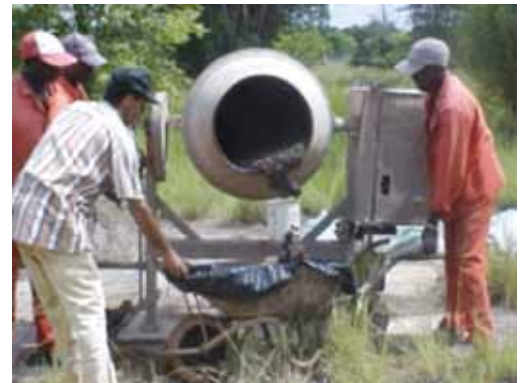
Discharging mixed emulsion
