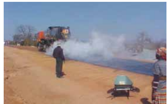
Hot bitumen temperature and toxic fumes
