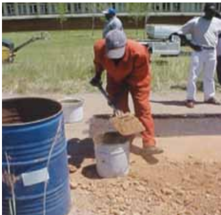
Batching aggregate, lime and cement
