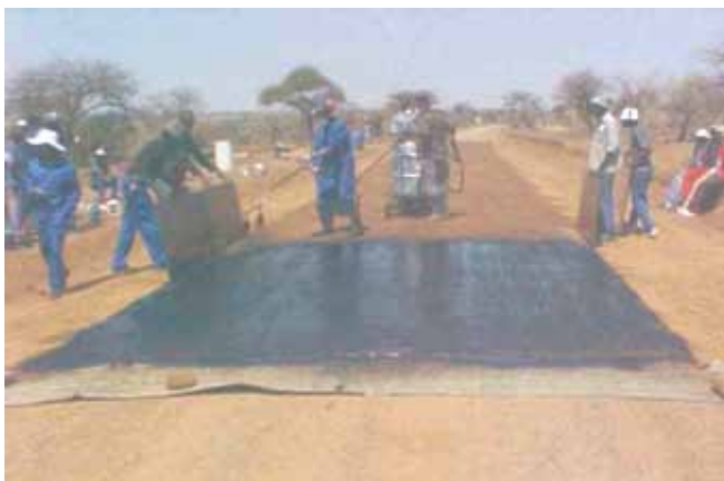
Spraying using protective screens and reinforced paper
