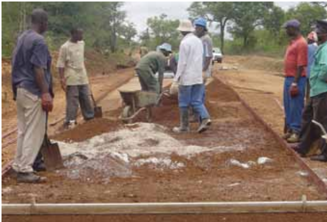
Lime stabilization in practice
