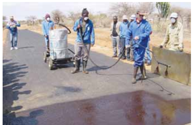
Spraying emulsion on an already primed surface
