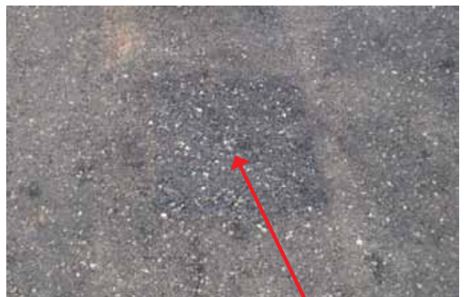
Finished "patch" hardly visible
