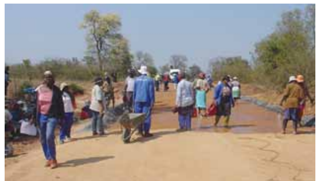
Watering the base Surface
