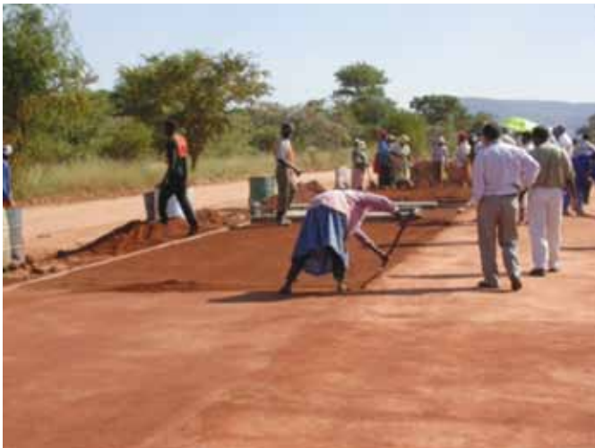
Spread and Compacted Base layer
