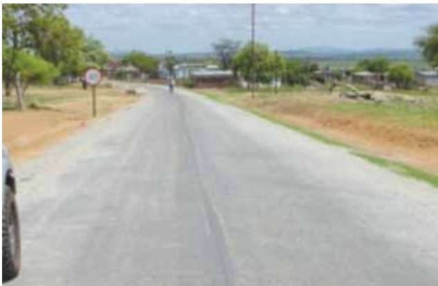
Sand Seal with Commercial Crusher Dust
