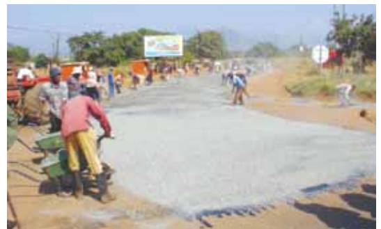
Slow spreading rate of aggregates by hand
