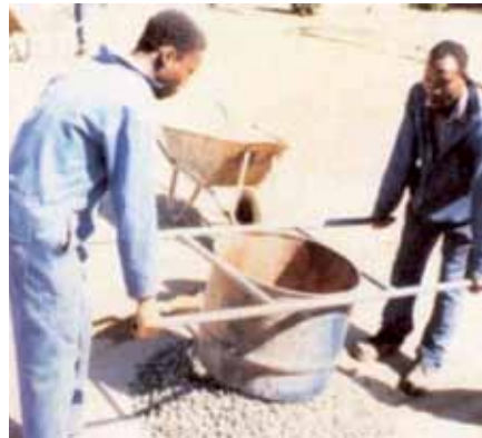
Figure 8-8: Spotting of aggregate
