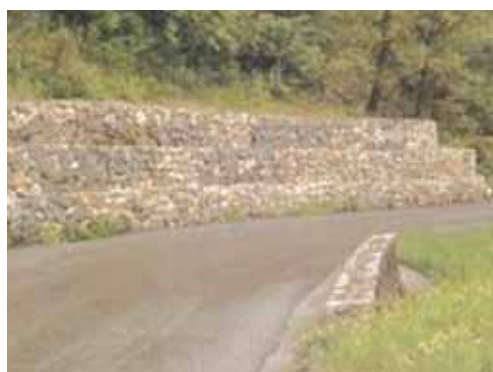
Gabions used as retaining wall for road side slope
