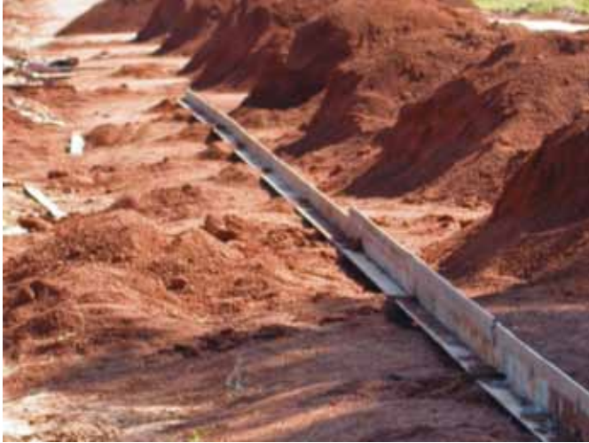
Setting out of Steel Shutters to retain Base Layer
