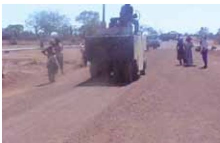
Compacting Otta Seal natural gravel
