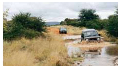
Roads without maintenance
