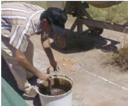
Mix remaining water and emulsion and add
