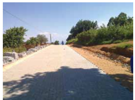
Packing of paving blocks
