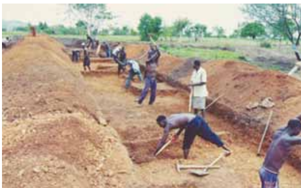
Excavation and stockpiling to create a loading bay
