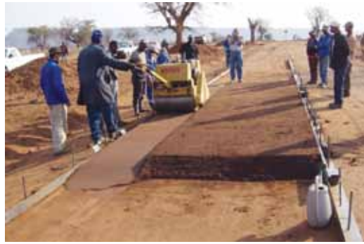
Compaction of ETB layer
