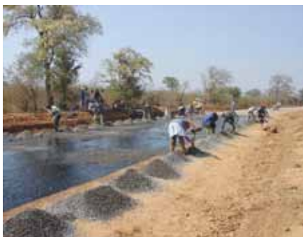
Spreading of aggregate by hand
