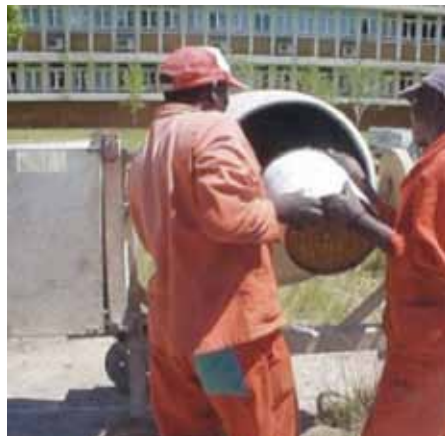
Feeding aggregate, lime and cement into mixer
