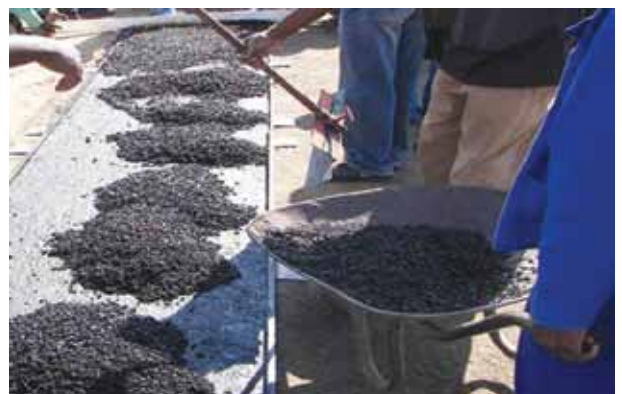
Spotting the asphalt
