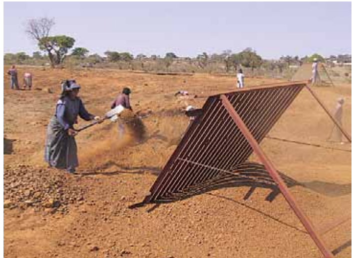
Sieving of natural aggregates at the borrow pit
