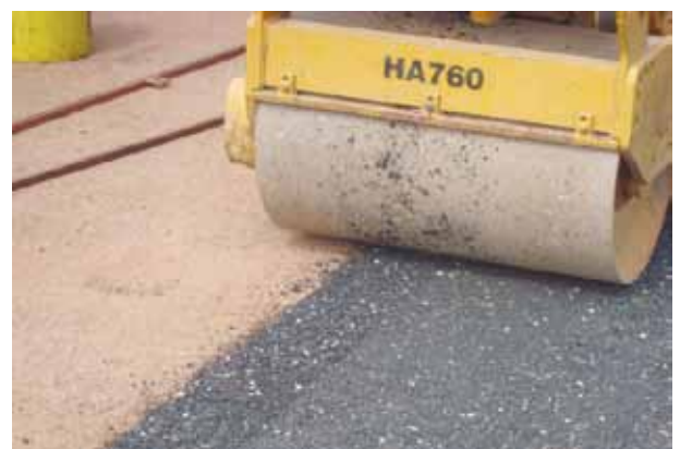
Compaction of asphalt
