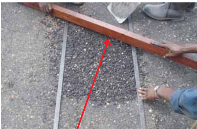
Screed the top
