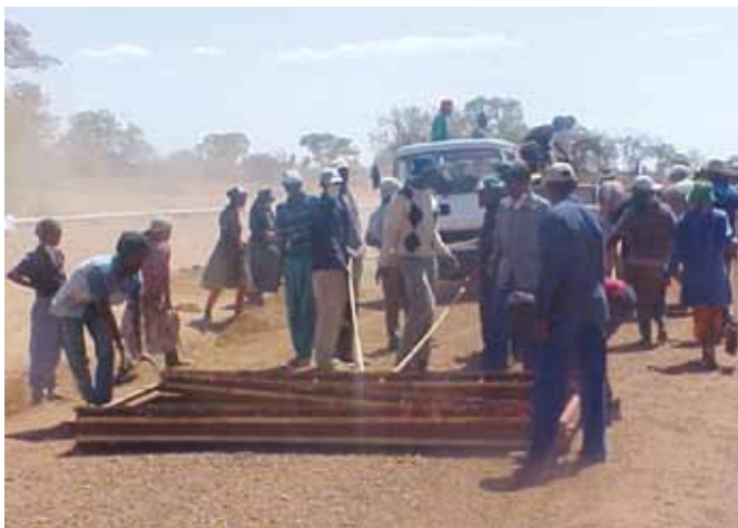
Using a drag broom to level spread natural gravel by hand
