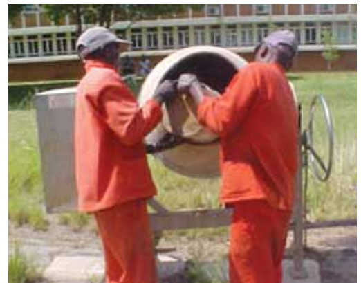
Adding aggregate to mixer
