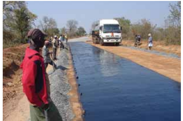
Spraying Bitumen by Bitumen Tanker
