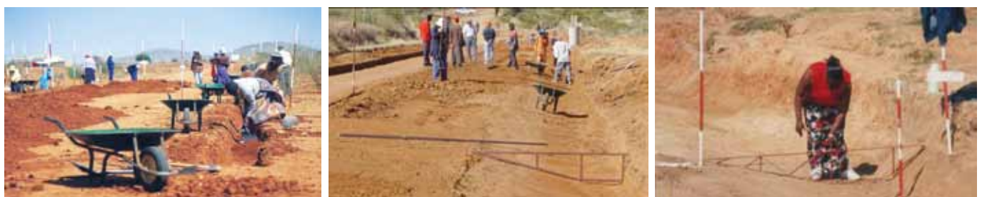
Constructing open drains using labour-based work methods
