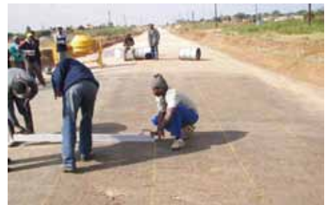
Marking position of guard rails
