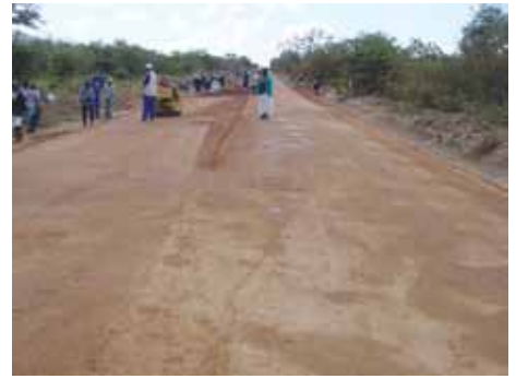
Compacted ETB layer
