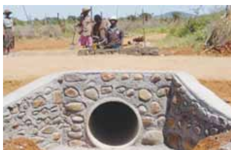
Stone pitched culvert wing wall
