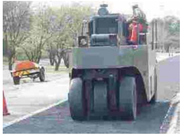
Compaction by a Pneumatic Roller
