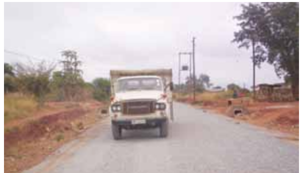
Loaded Tipper Trucks assisting in compaction
