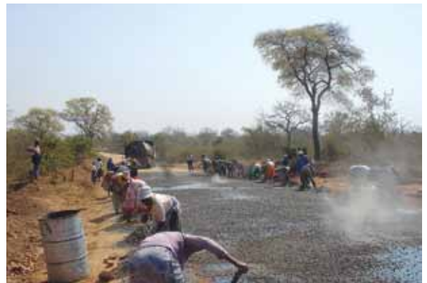
Aggregate spreading by Hand
