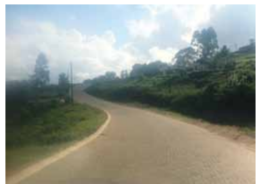
Completed block-paved sections
