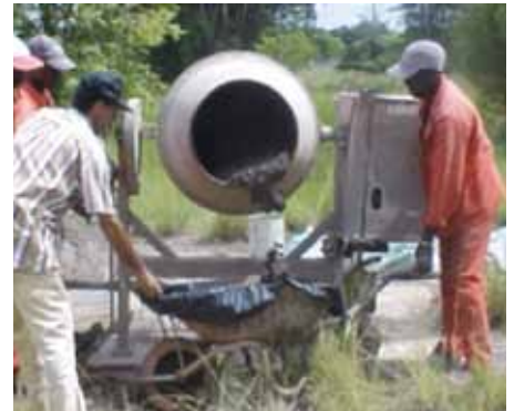
Discharging the mixed ETB
