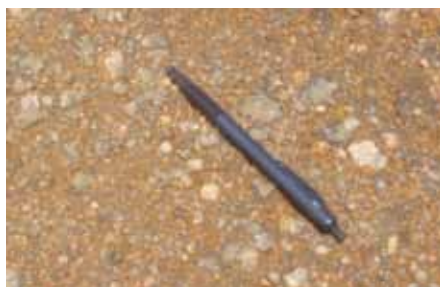
Compacted natural gravel Otta Seal
