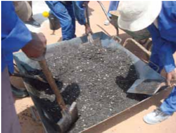
In-situ hand-mixing of asphalt
