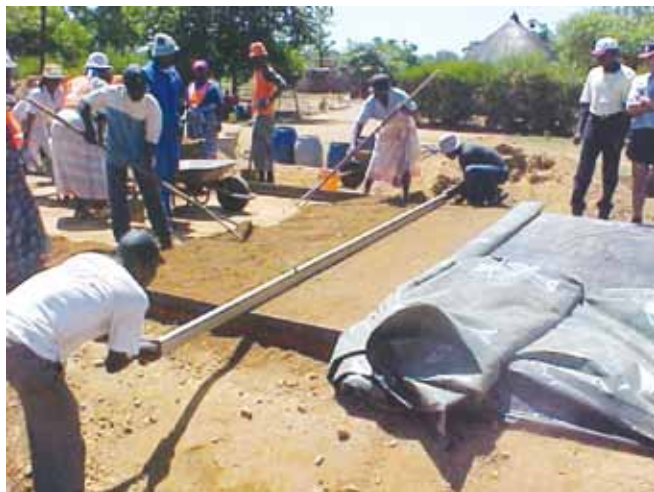
Use of plastic cover to prevent moisture loss
