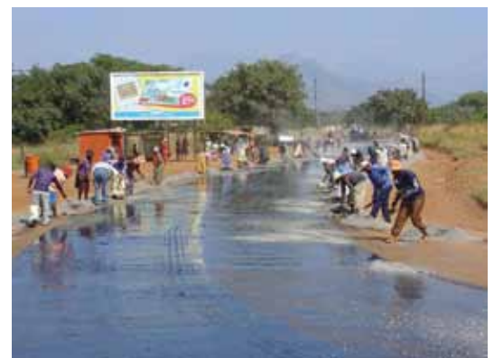
Hot bitumen temperature and toxic fumes
