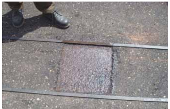
Area prepared for placing of asphalt
