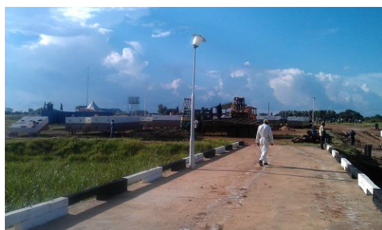
Namasale Ferry being assembled on site
