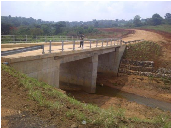
Kaichumu Bridge Completed
