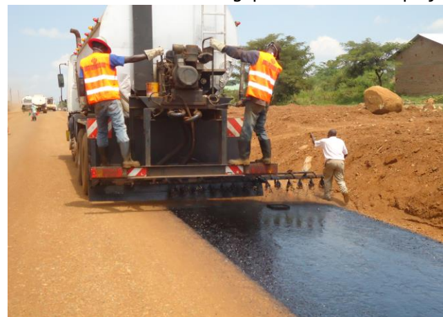
Tororo – Mbale Road Rehabilitation works
