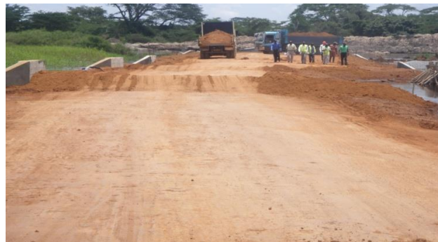
Bridge under construction
