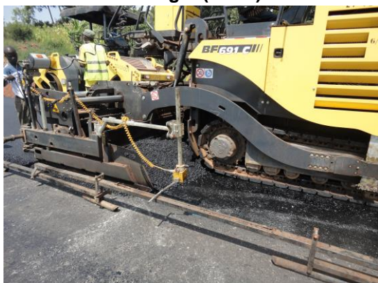
Malaba – Bugiri overlay using pavement recycling technology
