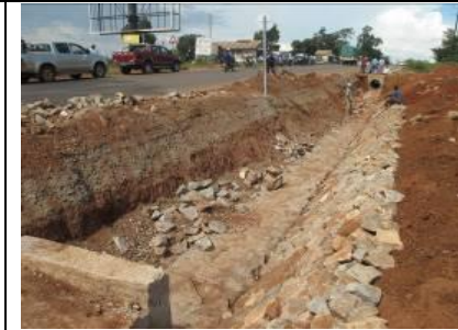
Repair of damaged lined drain at Iganga
