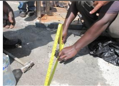
Measuring thickness of asphalt layer
