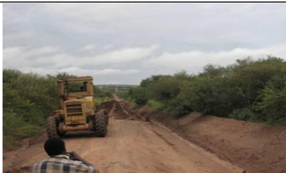
Poor quality clayey material dumped as fill material along fill sections
