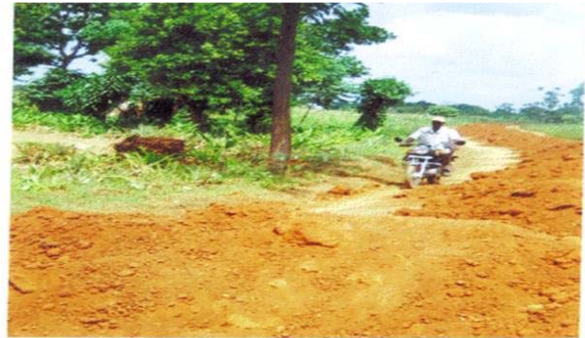
Figure 4: Unspread and Overstayed Murram - Kachocho Road being Under Rehabilitation
