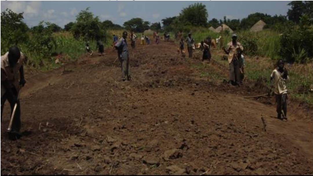
Figure 2: Labour-Based Activities in Apapai-Ogera Road in Serere County, Soroti District
